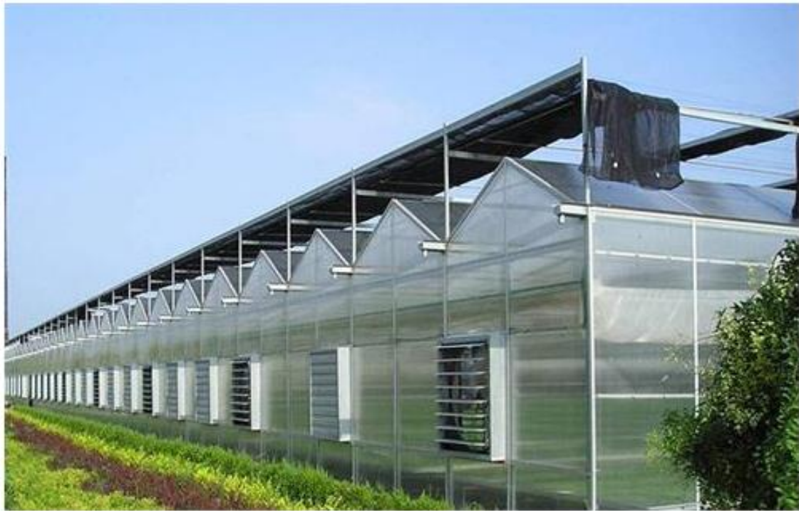
Figure 2.4 Greenhouse with glazing made of glass [16]
