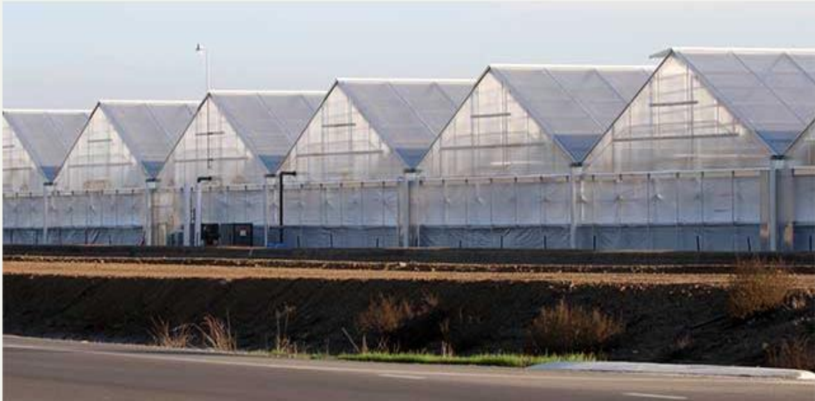
Figure 2.3 Greenhouse with a gable roof [14]
